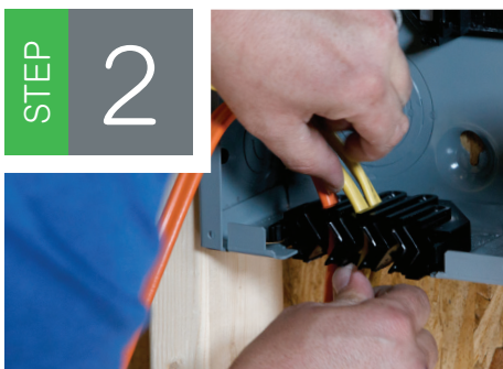
Slide the wire into the slot
