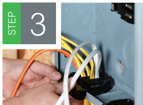
Snap on the Qwik-Grip shield when all circuits are installed
